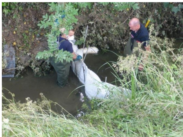
Photo 4 Custom-made barriers and filter systems for polluted small streams (source Cedre)
